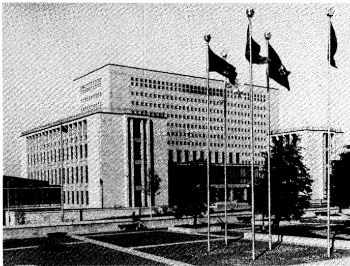
The Public Archives moved to its new location in 1967. ( Public Archives of Canada )
